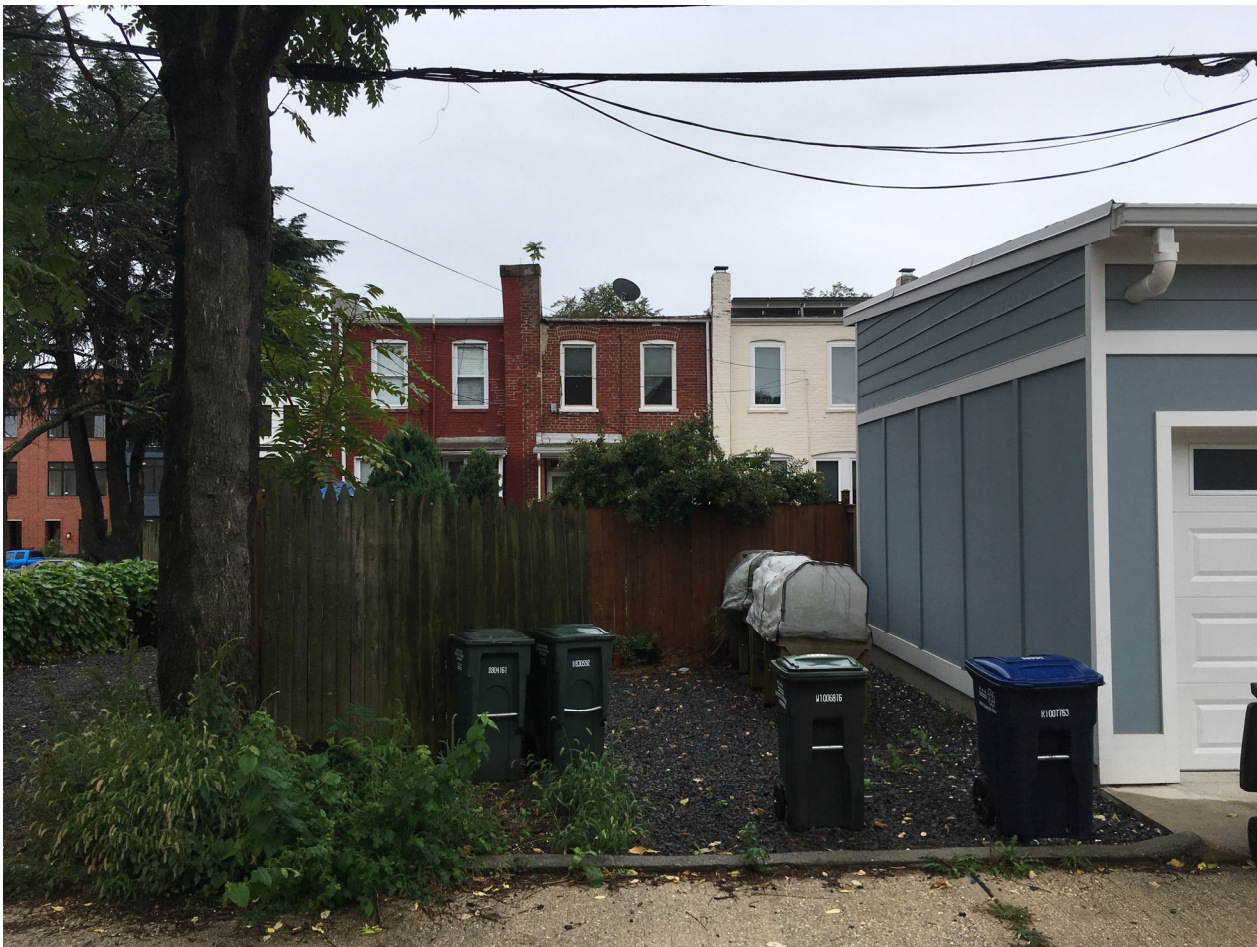
REAR VIEW FROM REAR ALLEY
