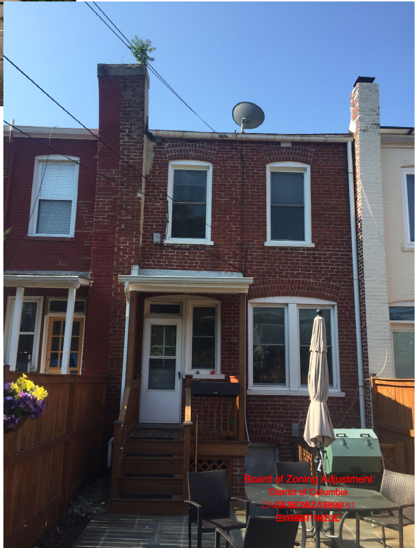
EXISTING REAR FACADE
