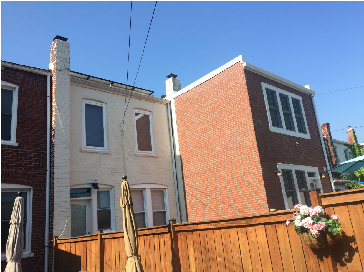
REAR VIEW LOOKING EAST
