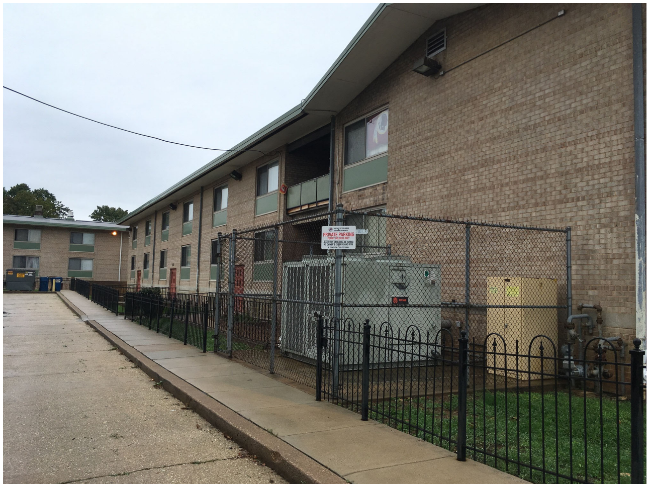
APARTMENT BUILDING TO THE NORTH AND EAST
