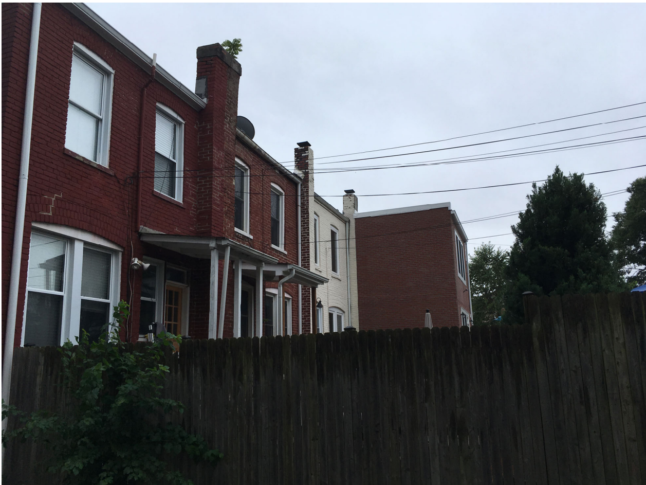
REAR VIEW FROM SIDE ALLEY (LOOKING EAST)
